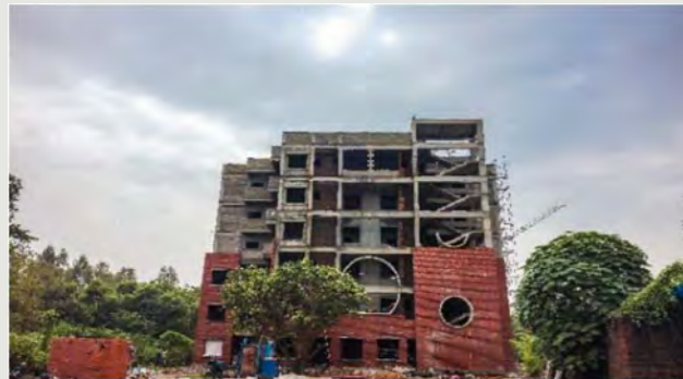
Students Hostel under construction
