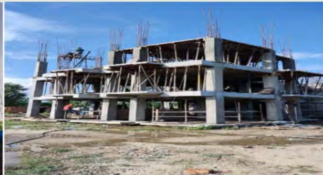
Staff Quarters under construction
