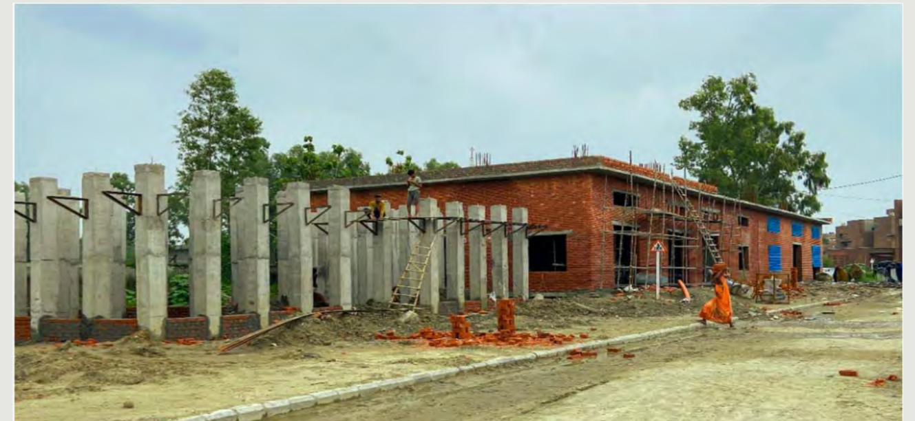
New HVAC Plant under construction
