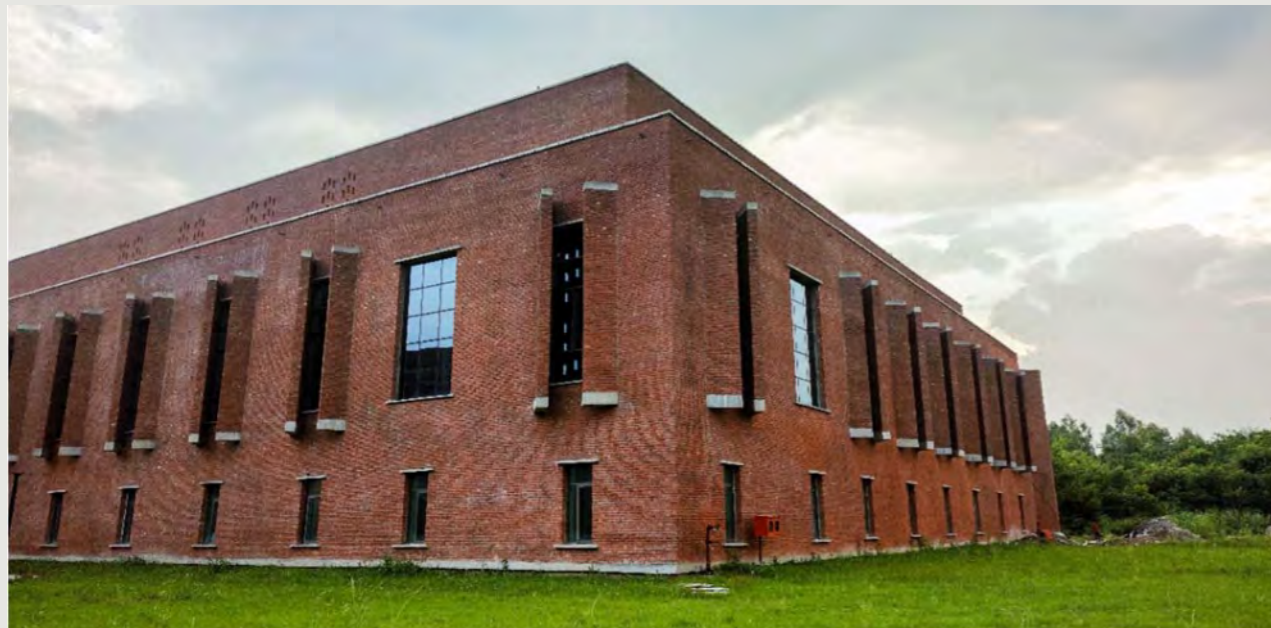
New Library Building under construction
